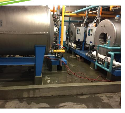
Hydroclave holding tanks found FULL with water backing up through the drainage system
